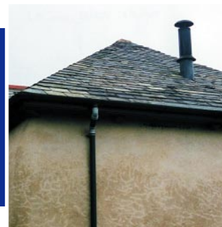
Unobtrusive metal flue painted black
